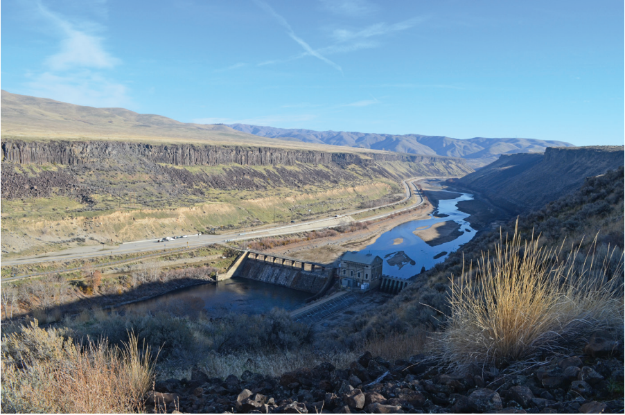
View of Diversion Dam and Boise River Canyon
